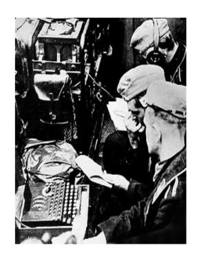
The Enigma machine looked like a typewriter in a wooden box. An electric current went from the keyboard through a set of rotors and a plugboard to light up the 'code' alphabet.
